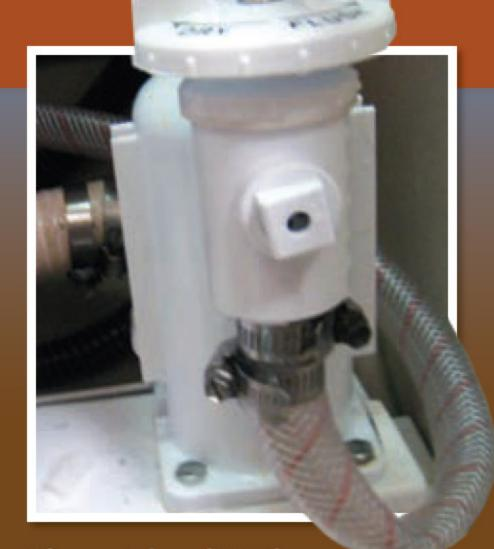
Clear, reinforced PVC hose, while fine for pressurized freshwater systems, is not a good choice for tight turns or suction-side applications, and it won't fight odors as well as a premium hose.
